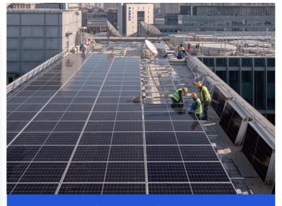
The photovoltaic systems installed on the roofs of Baidu Campus and Penghuan Building generate 1 million kWh of electricity annually, reducing carbon dioxide emissions by around 600 tons
